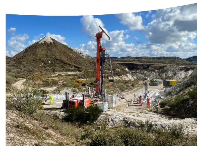
Cornish Lithium Reverse Circulation Rig at Trelavour, near St Austell
