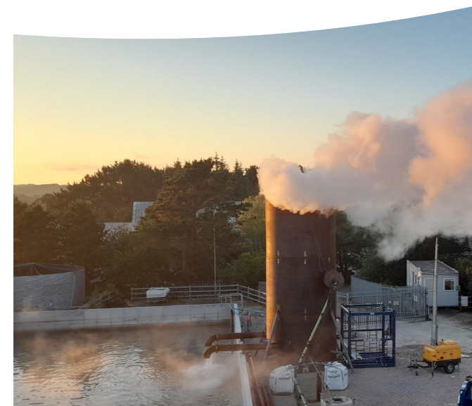
United Downs Deep Geothermal final testing phase
