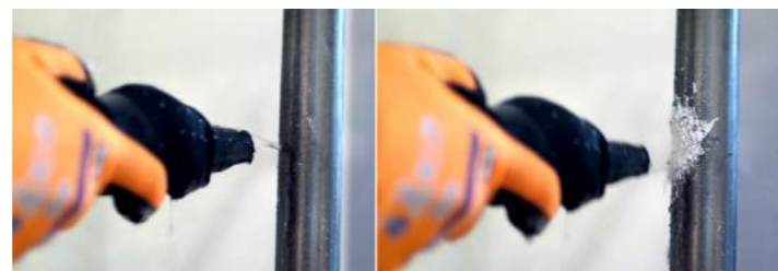
M3Spray sealing a water leak from a mild steel pipe
