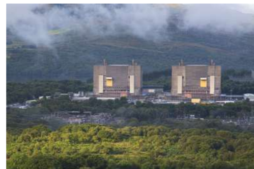
End state of Magnox reactors Graphite civil and research sites
