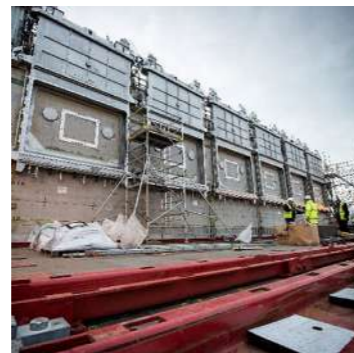
Pile Fuel Cladding Silo - Waste bunker retrieval project
