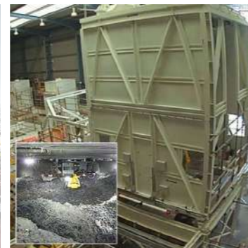
Berkeley Vaults - Waste bunker retrieval project
