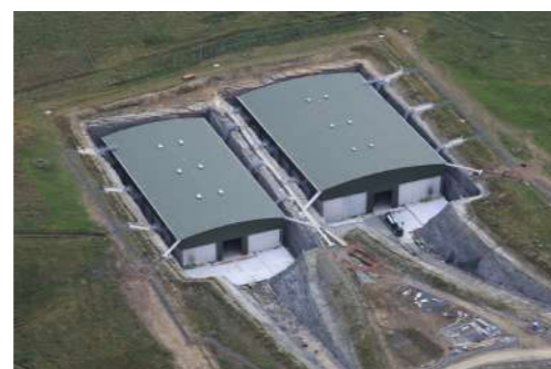
Near surface LLW engineered disposal facility at Dounreay Center of fast reactor United Kingdom
