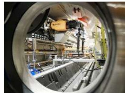
Fukushima Unit 2 DexterTM remote maintenance system in the boom containment cell.
