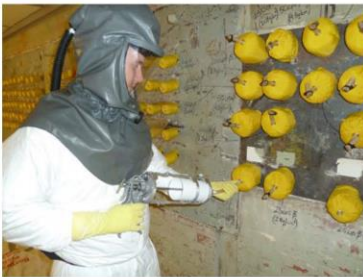
Foam cap-end installation at Harwell BEPO storage block
