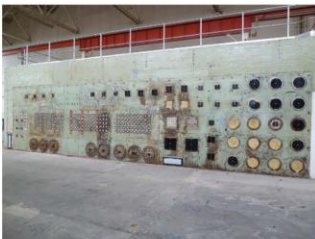
Harwell BEPO storage block on completion of SVI foam filling operation with 250 bespoke FOAMBAG™
