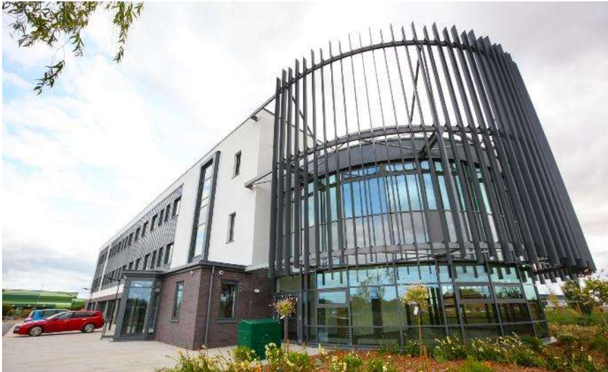
Somerset Energy Innovation Centre
