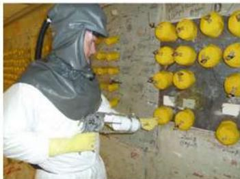
Foam cap-end installation at Harwell BEPO storage block
