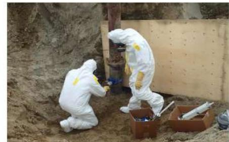
Canadian Nuclear Laboratories carrying out a pipe sealing operation on an active pipe using a bespoke FOAMBAG™ kit designed specifically for their project
